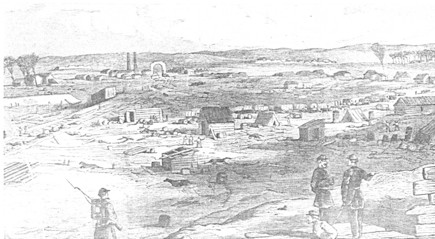
Contemporary view of Manassas Junction, Va.
